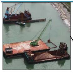
Placing sand blanket which acts as drainage layer
