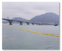
Installation of perimeter silt curtain
