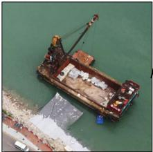
Laying geotextile for seabed protection
